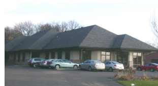
The Bridge's new home!
